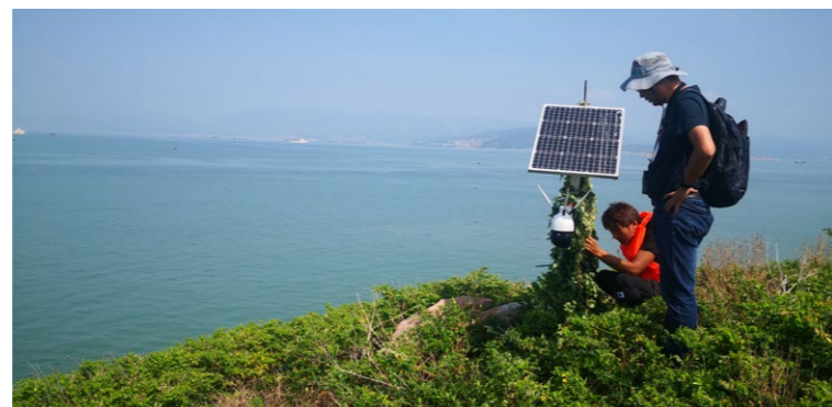
■ Installing solar-powered monitoring cameras
